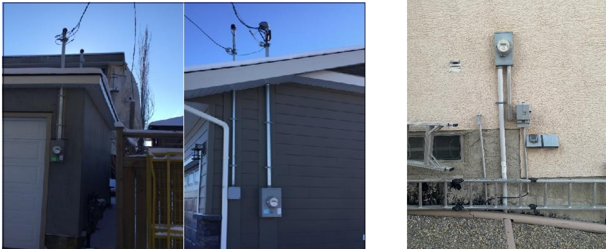
Figure 2: Overhead vs Underground service
